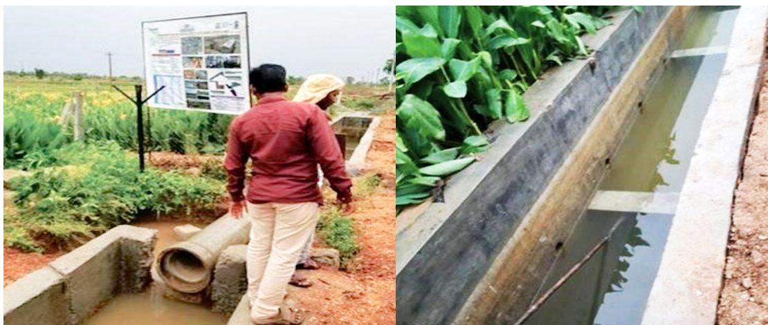
Figure 6: Equalization Chamber and Aerobic Baffled Reactor
