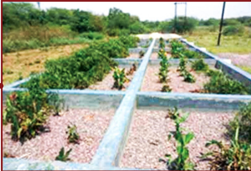
Figure 4: Phytorid Plant Constructed at Dhorka, Haryana
