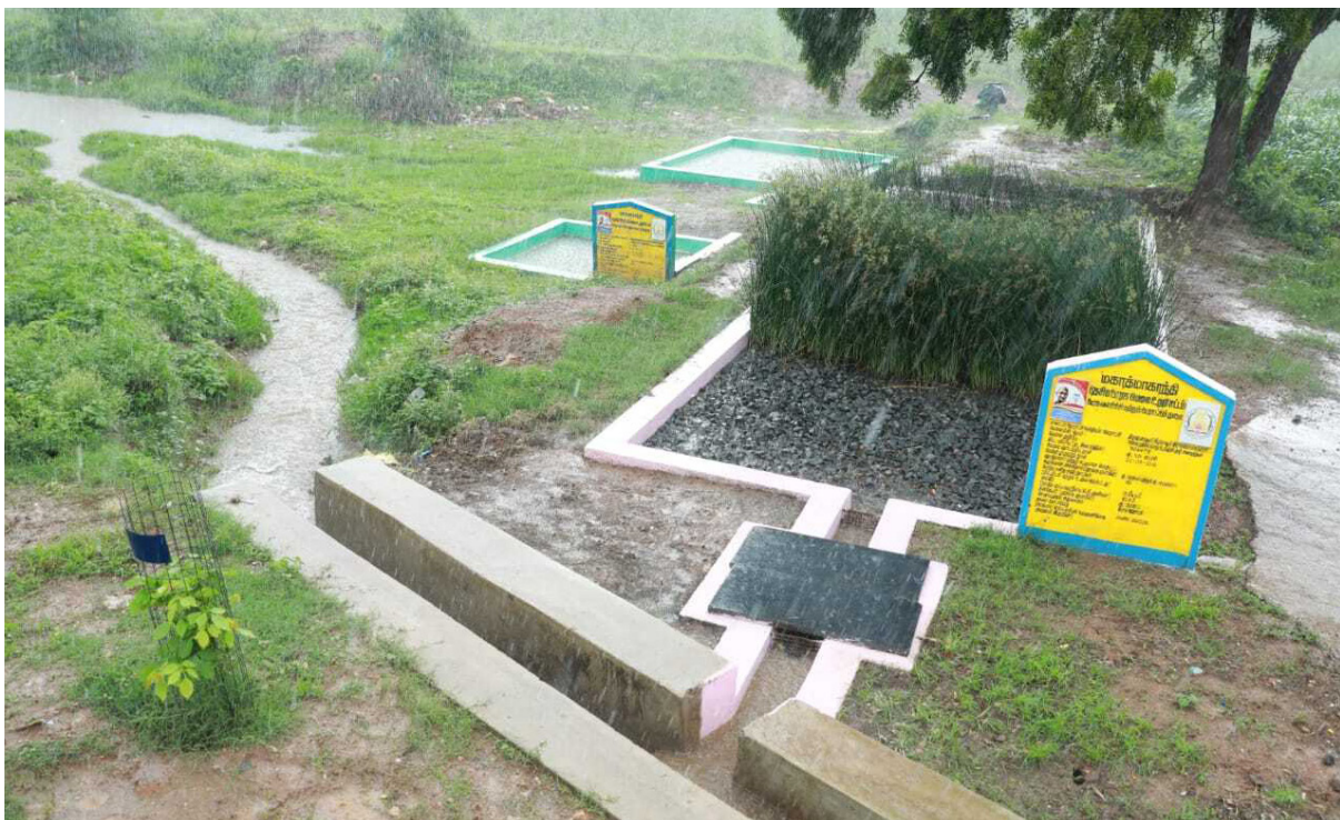
Figure 5: Community Horizontal Filter System
